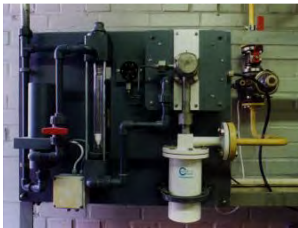
MR 50 RC Vacuum System additionally equipped with motor valve
